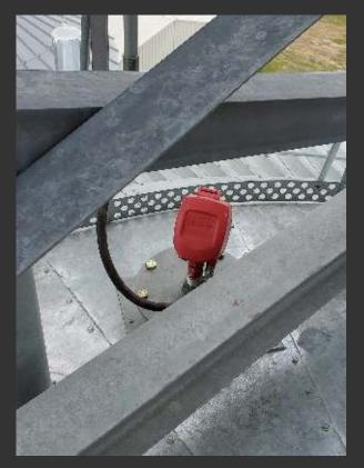
About five years ago, the mill added 3DLevelScanners to several of the bins where a higher level of inventory accuracy was needed in feedstuffs that piled unevenly in silos.
