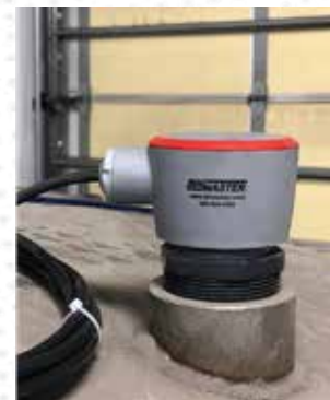
CNCR-130 installed on a fertilizer bin
